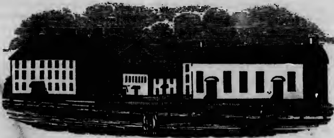
Shaker Buildings in New Lebanon.
